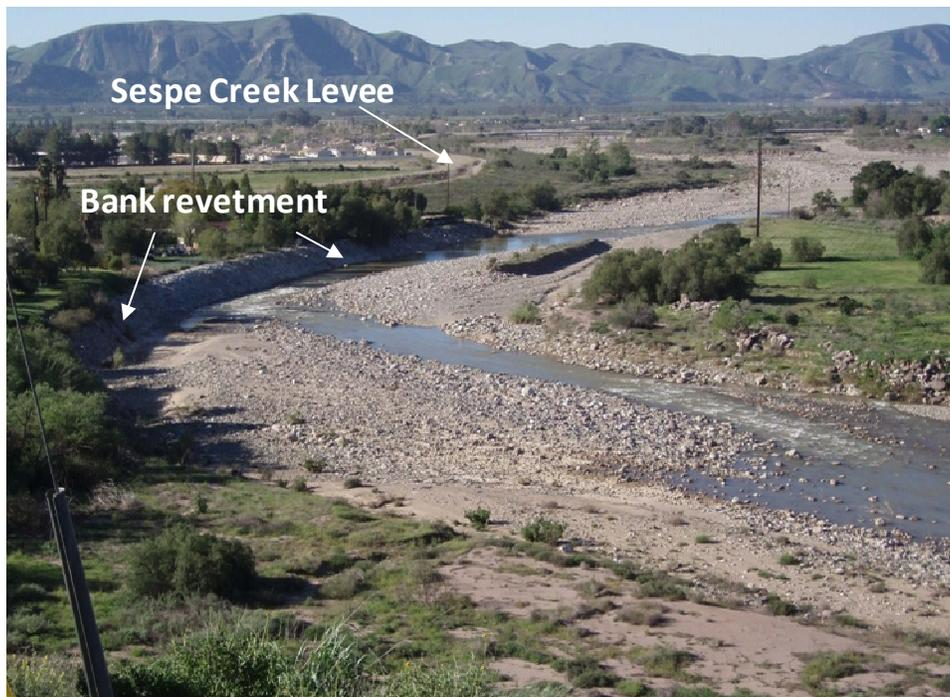
Figure 2-38. View of the concrete-rock bank revetment structure located along the left bank upstream of the Sespe Creek Levee in the Fillmore reach. View is looking downstream.
