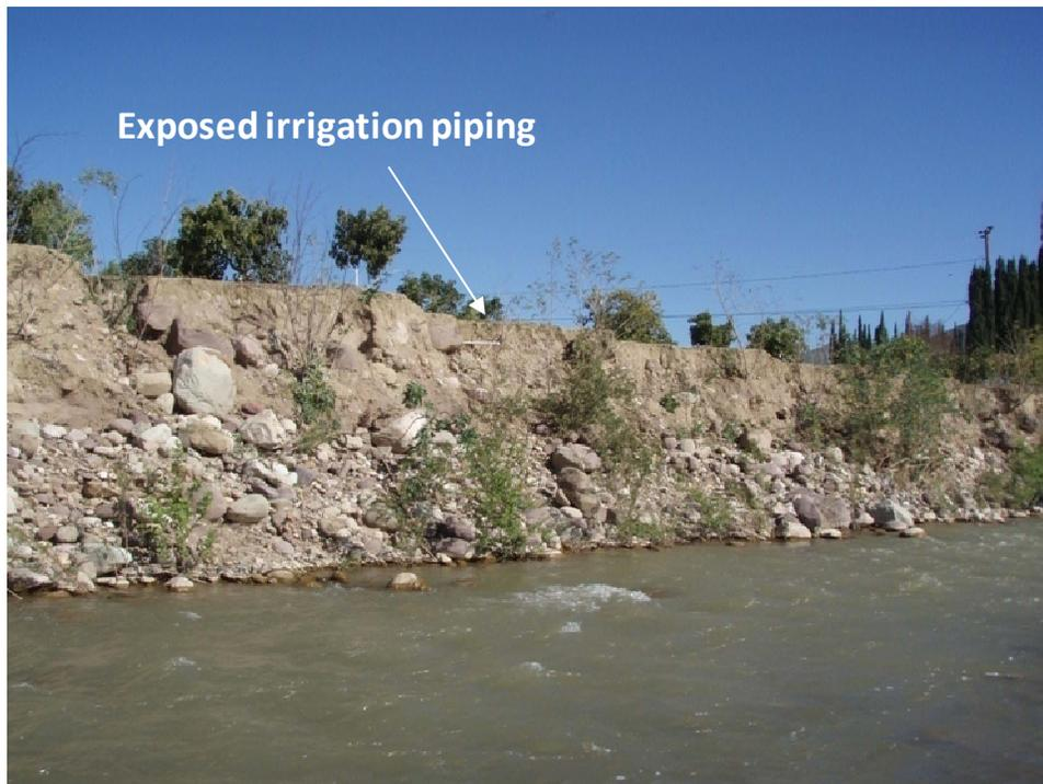
Figure 2-40. View of exposed irrigation piping and fruit tree roots at actively eroding right bank opposite the upstream end of the Sespe Creek Levee in the Fillmore reach.
