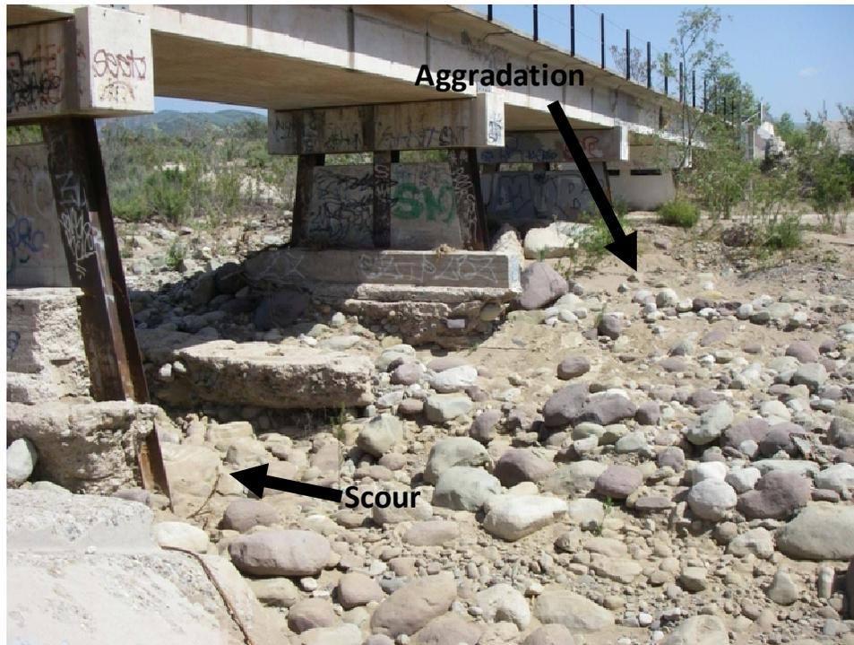
Figure 2-41. View of scour and deposition on either side of a bridge support for the Southern Pacific Railway bridge immediately upstream of the Old Telegraph Road Bridge on the east fork (overflow) of Sespe Creek in the Fillmore reach.
