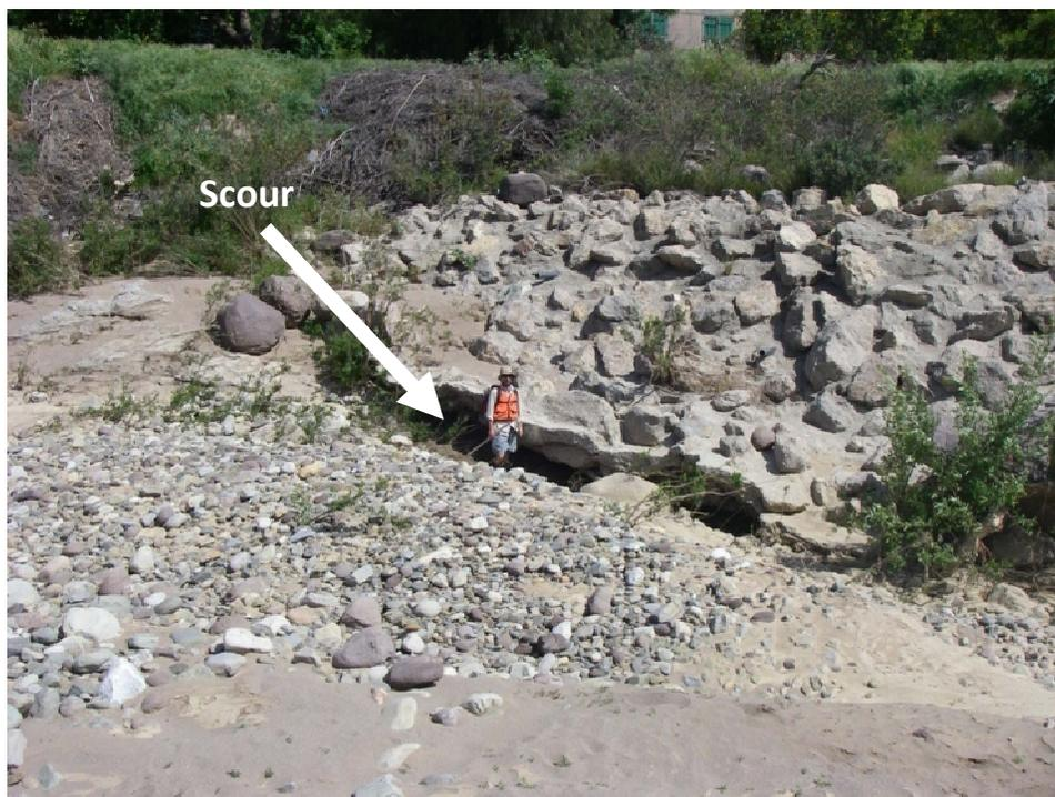
Figure 2-39. View of scour at the upstream end of the bank revetment structure located along the left bank upstream of the Sespe Creek Levee.
